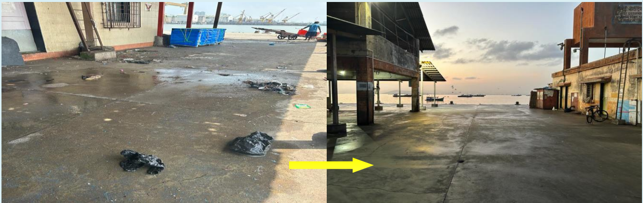
Cleaning of New Ferry Wharf harbour on daily basis by MbPA
